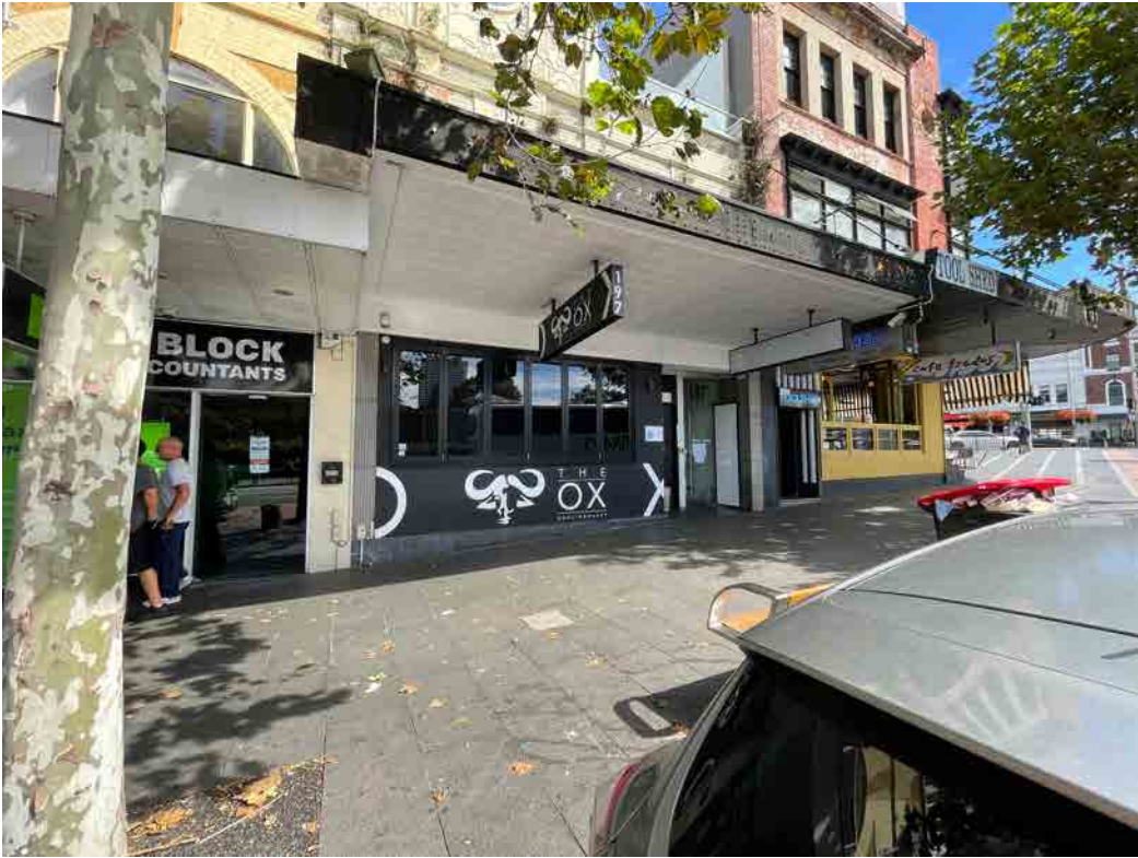
View of the subject site 191 - 199 Oxford Street
