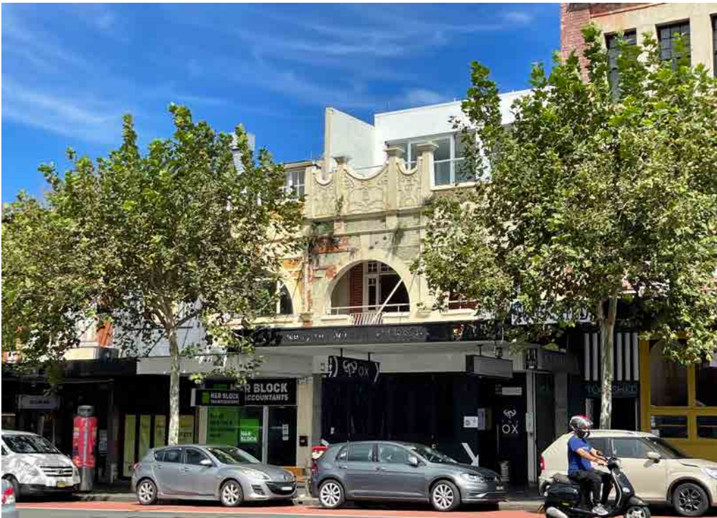
View of the subject site from Oxford Street
